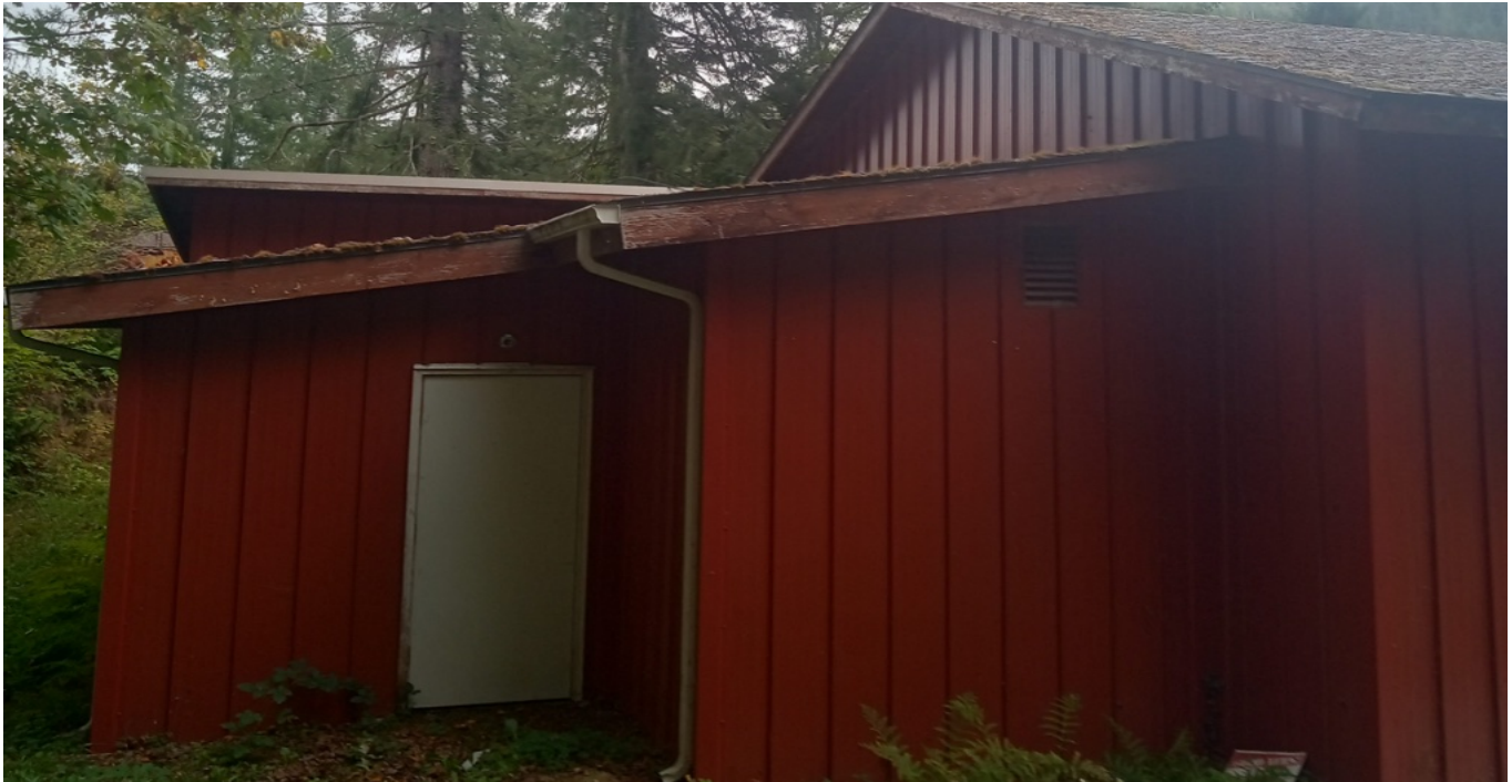
Figure 3: NORTH WEST SIDE OF BUILDING
