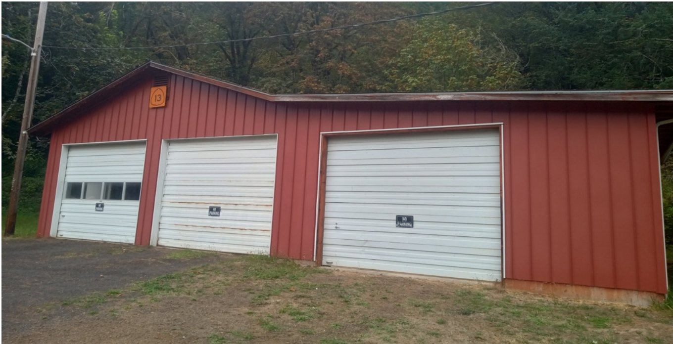
Figure 1: SOUTH FACING WALL
